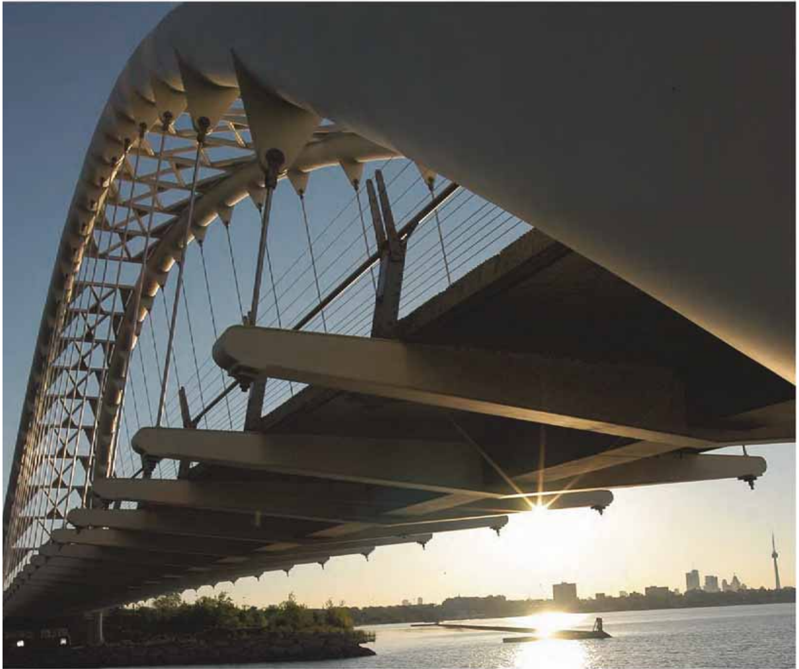
Humber River pedestrian bridge
